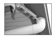
**Step 11.** Apply silicone sealant to the gutter pot to ensure that there are no leaks.
