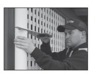
**Step 3.** Using a PVC saw or hacksaw, cut the downpipe horizontally across the top line. You will then need to remove the top section of your downpipe. You may need to detach the top of the downpipe from the gutter's running outlet or other connector.
