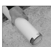
**Step 8.** Apply PVC cement to the bottom end of the top section of the downpipe.
