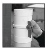
**Step 6.** Insert the Bushfire Buddy onto the bottom section of the downpipe and rotate so that the Bushfire Buddy lever is positoned where it is easily accessible.
