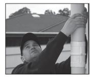
**Step 9.** Reinstall the top section of the downpipe to the joiner at the top of the downpipe and insert into the top of the Bushfire Buddy.
